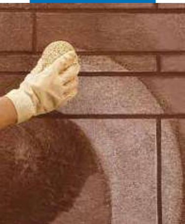
Cleaning and finishing the tile joints with a sponge
